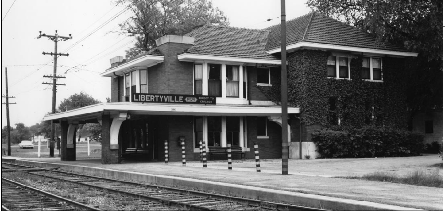
▲ Samuel Insull's trip was a 2 ½-mile drive north on Milwaukee Avenue from his mansion to the North Shore station shown here on May 27, 1962.— Joe Pierson photo
