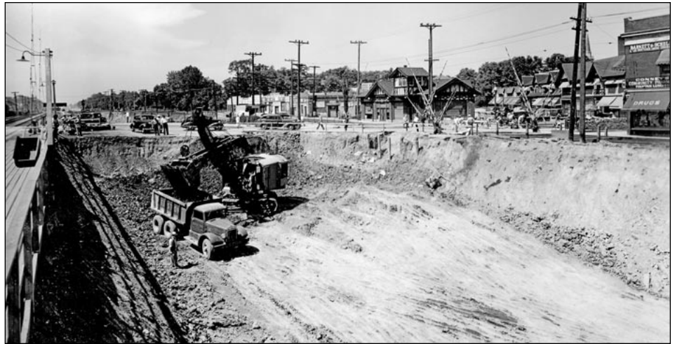
▼ Excavation is well underway south of Elm Street on July 27, 1939. This width of the cut is necessary to provide for the low-level platforms for C&NW and North Shore's high-level platforms.— Courtesy of Winnetka Historical Society
