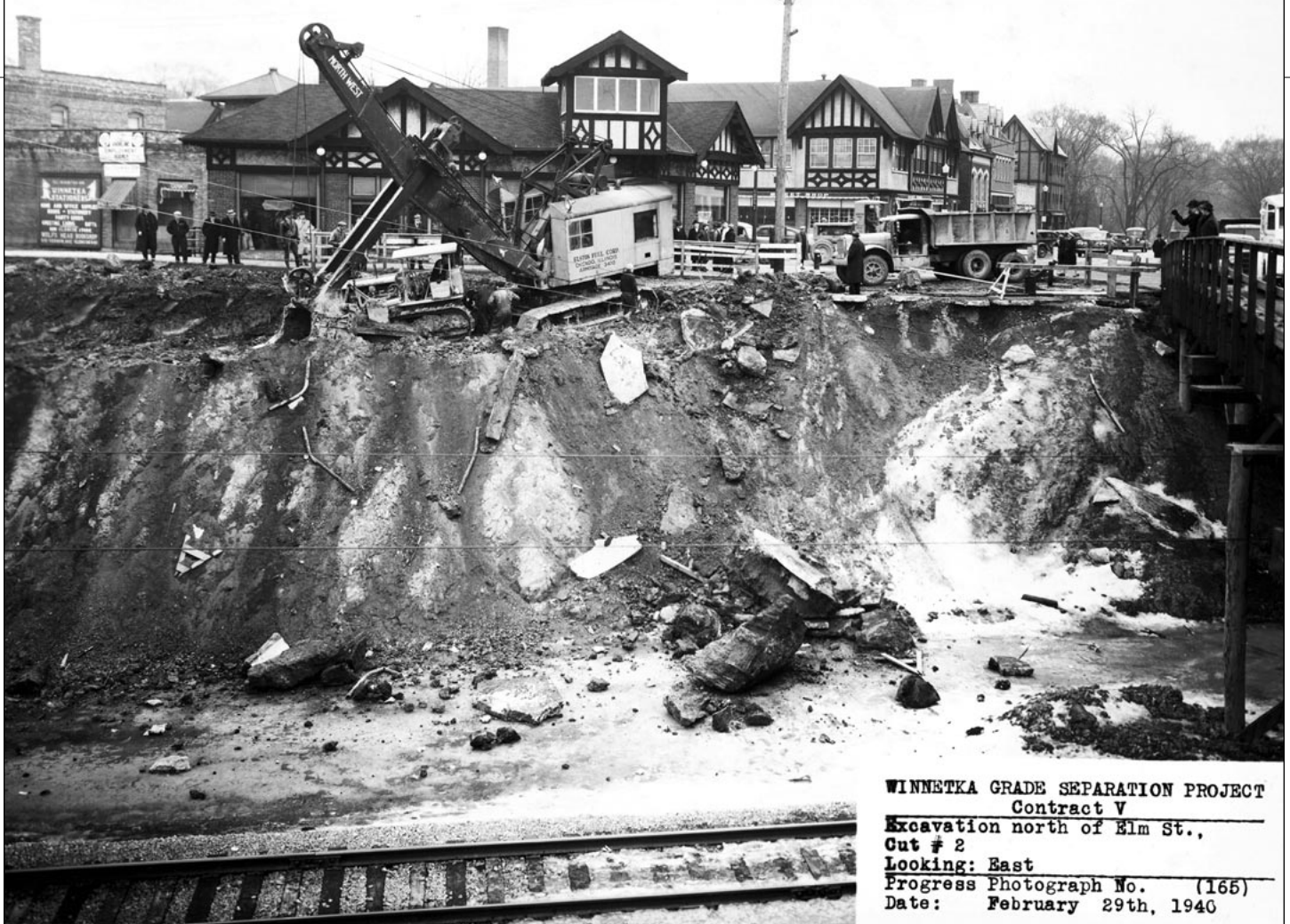
▲ On February 29, 1940, North Shore's right-of-way is being excavated to provide room for the new Elm Street station.— Courtesy of Winnetka Historical Society
