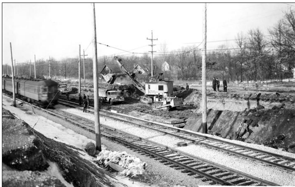
▲ On February 15, 1940, this southbound is running on what will become the permanent C&NW main lines. North Shore's infrastructure has been removed from its right-of-way in preparation for construction of the new infrastructure. We are looking north from Woodland Avenue, two blocks north of Winnetka Avenue in the transition from the cut to the elevation.— Courtesy of Winnetka Historical Society
