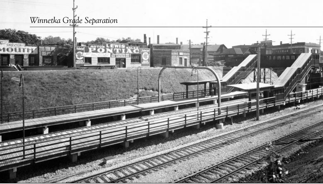
▲ On September 25, 1940, the Elm Street station is complete and appears to be in service. There is no evidence of trolley wire over what will become C&NW's permanent new main line tracks. This leads us to believe that North Shore's temporary use of the C&NW tracks was for approximately 10 months.— Courtesy of Winnetka Historical Society
