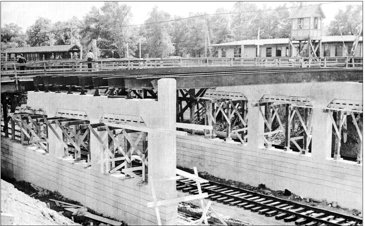
▲ Contract XI covered the construction of permanent highway bridges. Deckert and McDowell, Contractor. Total cost—$250,000. The continuous beam design combines simplicity of construction, economy and attractive lines. This view shows construction of the Elm Street bridge. Note temporary North Western Winnetka Station in background.— Courtesy of Northwestern University
