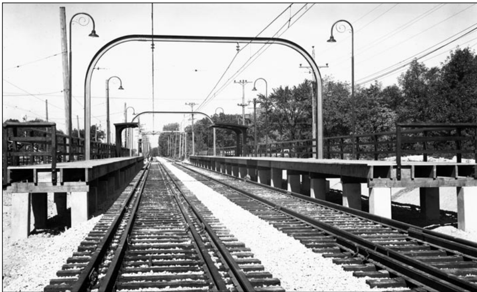
▲ By September 26, 1940, the construction work on the North Shore is completed. We are looking north at the Harbor Street station. Harbor Street is the first level grade crossing marking the north end of the grade separation project. Considering that North Shore had no freight service on its Shore Line route south of Elm Place at the north end of downtown Highland Park, the gauntlet tracks are curious. Indian Hill was a low-level platform. All stations from Willow Road north to Harbor Street were built with high-level platforms and gauntlet tracks.— Courtesy of Winnetka Historical Society
