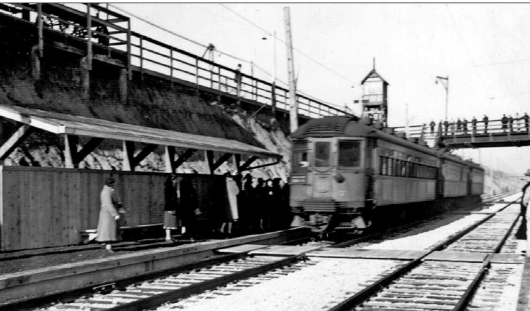
▲ On November 28, 1939, 11 months after construction started, the first southbound North Shore train is operating on what will become the C&NW's permanent right-of-way. Most likely this train is at Elm Street.— Courtesy of Winnetka Historical Society
