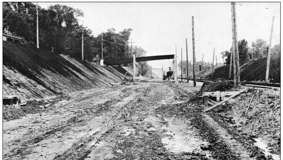
▲ Contract XI covered the construction of permanent highway bridges. Deckert and McDowell, Contractor. Total cost—$250,000. The continuous beam design combines simplicity of construction, economy and attractive lines. This view shows construction of the Elm Street bridge. Note temporary North Western Winnetka Station in background.— Courtesy of Northwestern University
