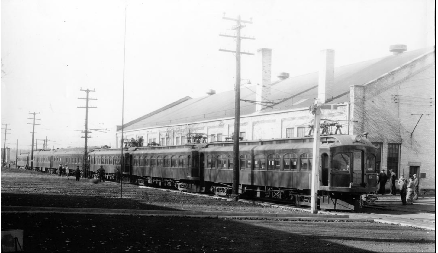
▲ In 1925 this Lake Shore special train is stopped at Shops on an eastbound trip. Behind the three motor cars are two Chicago & Alton Railroad dining cars. Lake Shore did not provide dining car service. We are wondering if this is an inspection trip of the newly acquired railroad for the Insull management team and friends.—Calvert Studio photo for the railroad, William C. Janssen Collection
