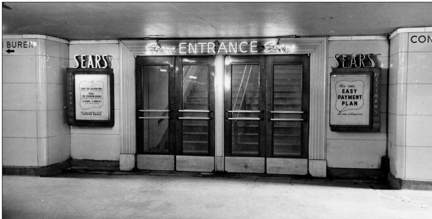
▲ Station mezzanines were designed to allow connections to adjacent buildings through the strategic placement of structural supports and bulkheads, allowing sections of wall to be more easily removed to make the connections. Each connection looked unique, however, evoking the style and design of the store or tenant. Sears' flagship store had a direct connection to the Van Buren-Congress mezzanine, seen in 1956. —CTA photo
