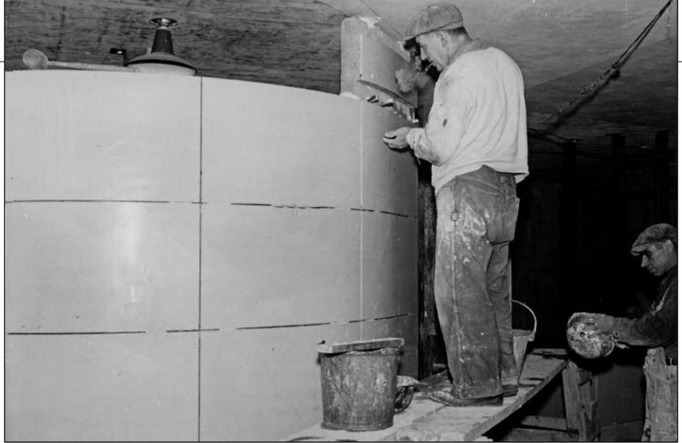
▲ Masons work to install structural glass panels in a downtown station mezzanine on July 30, 1942. The 18-inches by 31-inches structural glass panels were delivered clipped to a concrete block backing by means of zinc clips extending completely around the perimeter of the glass block. The edges of the glass were beveled so that the zinc clips would hold the glass to the concrete blocks more firmly. These blocks were laid much as a bricklayer lays bricks but with greater accuracy. —CTA Collection
