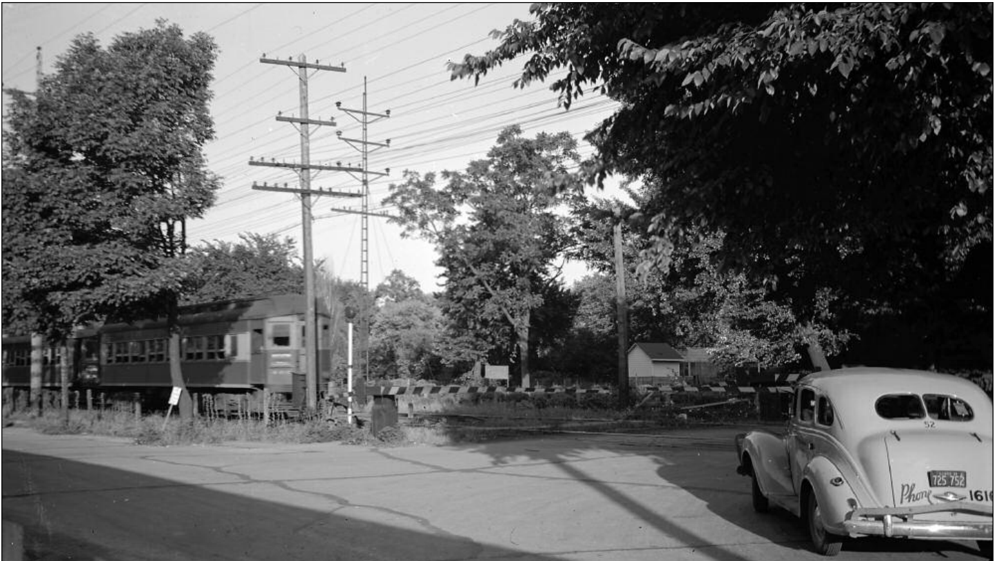
▲ In June 1946 car 417 is heading an eastbound train near Park Boulevard. The circular concrete building on the C&NW houses the automatic train control system technology. The slow sign at the far left of the image was the “set-em up point” for braking for the Main Street station stop. On the CA&E speed restrictions were “observed more in the breach than in the observance.” The trains would decelerate from to their station stop in 2-1/2 blocks. Usually the gates at Main Street were not all the way down when the “Cannonball” entered the Main Street crossing. ▼ Grade crossing protection consisted of manually operated four quadrant gates with a street bell that can be seen just in front of the train. Outside of the image to the right was a set of crossing flashers on the south side of the track. This westbound train is approaching the Forest Avenue crossing and the cab is turning off of Stewart Avenue. —Two photos Frank Krejcik, Walter Keevil Collection
