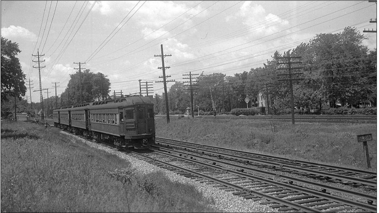
▲ In June 1946 car 417 is heading an eastbound train near Park Boulevard. The circular concrete building on the C&NW houses the automatic train control system technology. The slow sign at the far left of the image was the “set-em up point” for braking for the Main Street station stop. On the CA&E speed restrictions were “observed more in the breach than in the observance.” The trains would decelerate from to their station stop in 2-1/2 blocks. Usually the gates at Main Street were not all the way down when the “Cannonball” entered the Main Street crossing. ▼ Grade crossing protection consisted of manually operated four quadrant gates with a street bell that can be seen just in front of the train. Outside of the image to the right was a set of crossing flashers on the south side of the track. This westbound train is approaching the Forest Avenue crossing and the cab is turning off of Stewart Avenue. —Two photos Frank Krejcik, Walter Keevil Collection
