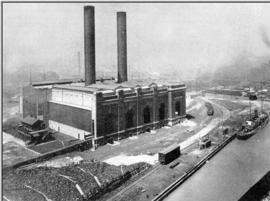
Fisk Street Station as it appeared while under construction in 1903. The general construction is of steel covered with red pressed brick and ornamented with heavy cut Bedford stone. *Photo from The Sargent & Lundy Story*
