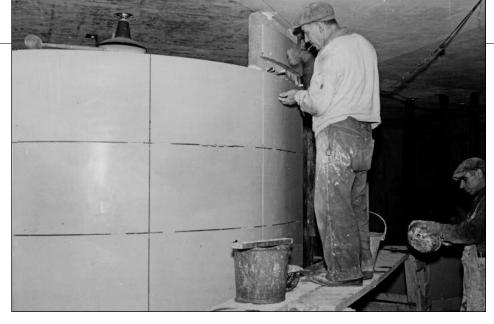
▲ Masons work to install structural glass panels in a downtown station mezzanine on July 30, 1942. The 18-inches by 31-inches structural glass panels were delivered clipped to a concrete block backing by means of zinc clips extending completely around the perimeter of the glass block. The edges of the glass were beveled so that the zinc clips would hold the glass to the concrete blocks more firmly. These blocks were laid much as a bricklayer lays bricks but with greater accuracy. -CTA Collection
