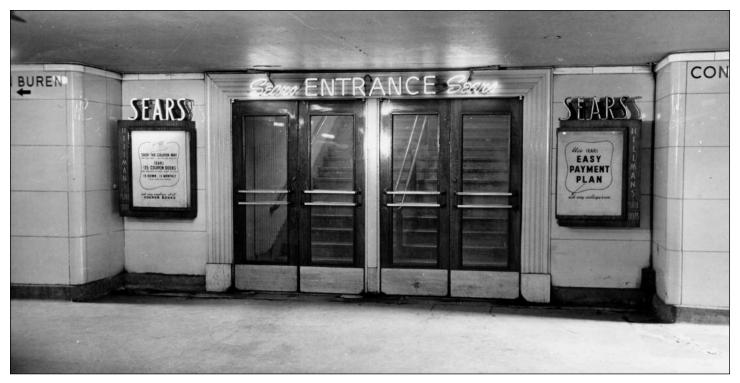
▲ Station mezzanines were designed to allow connections to adjacent buildings through the strategic placement of structural supports and bulkheads, allowing sections of wall to be more easily removed to make the connections. Each connection looked unique, however, evoking the style and design of the store or tenant. Sears' flagship store had a direct connection to the Van Buren-Congress mezzanine, seen in 1956. —CTA photo
