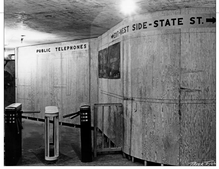
▲ In early 1942, the Jackson-Van Buren mezzanine was outfitted with turnstiles, dummy plywood walls and pillars for experimentation and study by engineers and designers. Several types of exit turnstiles were studied. False walls were erected to emulate the draft architectural designs, down to drawing the outlines of telephone booths and concession windows and applying paper lettering on the walls. —CTA Collection
